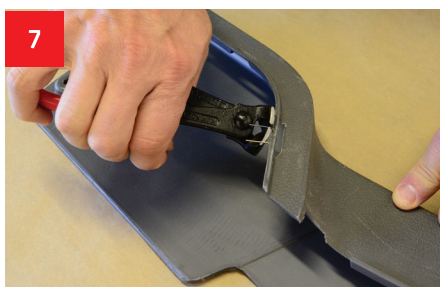
7 Any protruding ends of the staples should be cut using a cutter.
